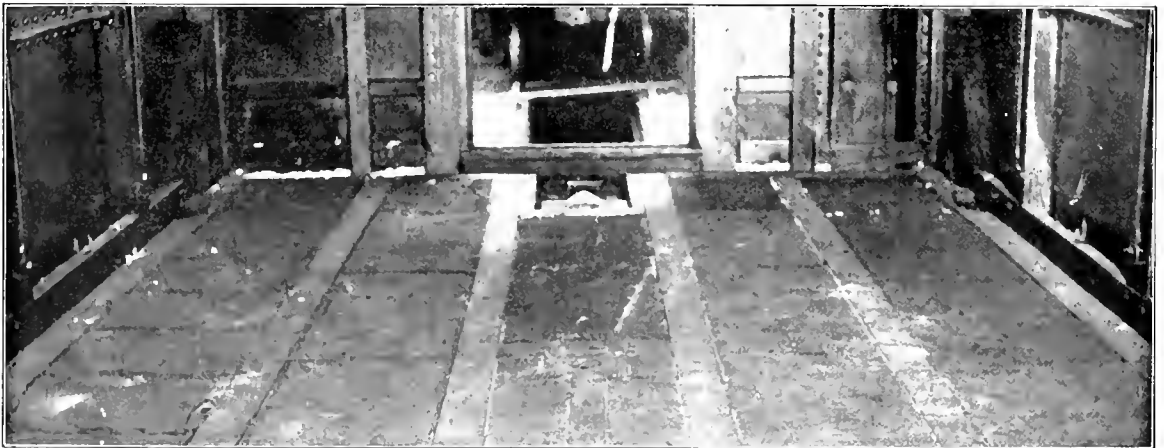
Tucork Floor Insulation in Place
